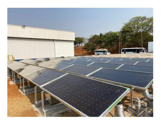
PepsiCo's partner supplier for the installation of thermosolar plants at the Feira de Santana and Sete Lagoas plants is TVP Solar, a Swiss company specialized in thermosolar technology with state-of-the-art solutions, with high vacuum solar thermal collectors and without mirrors, based on a patented technology.
